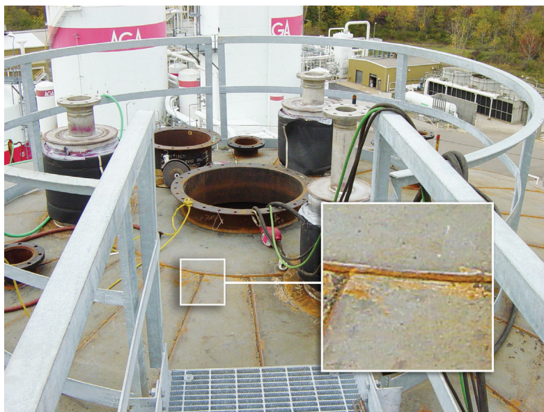
Figure 9. Dome roof weld for purge gas container for a LIN/LOX tank under construction indicating surface profile.
